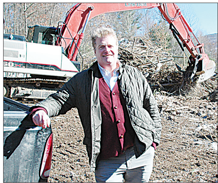
Lex Heslin oversees work on his property while John Zeh is working the excavator, clearing a former bungalow colony just up the hill from the old Homowack. Lex says the acreage being cleared will host solar panels, vertical wind turbines and a shallow geothermal system, all of which will be used to power the resort (with extra left over to return to the grid).
